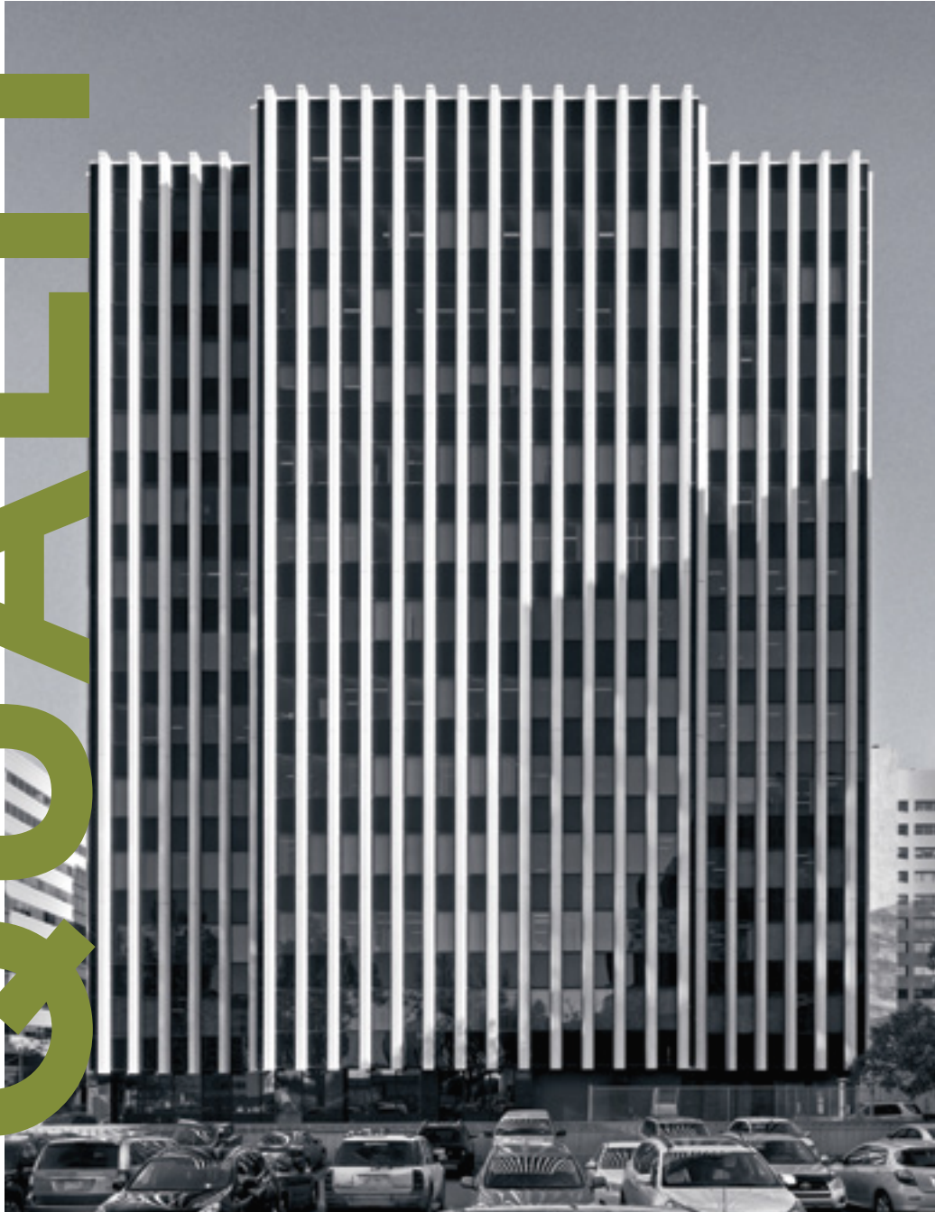
PETROLEUM PLAZA, EDMONTON, AB
